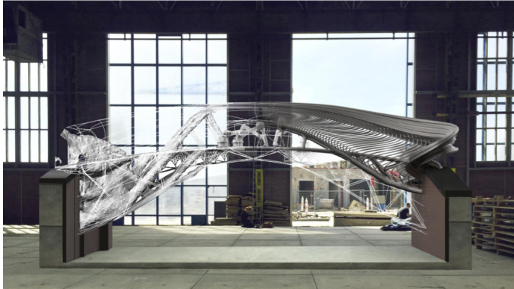
Figure 1—Generatively Designed Bridge in Partnership with MX3D for Robotic Fabrication (Courtesy of Autodesk)
